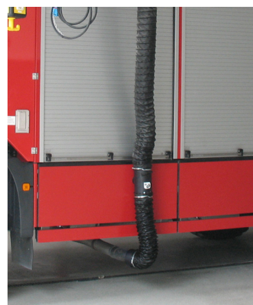
Magnetic-connected exhaust nozzle in suspended hose.
