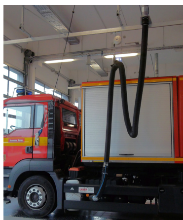
Pneumatic nozzle with suspended hose.
