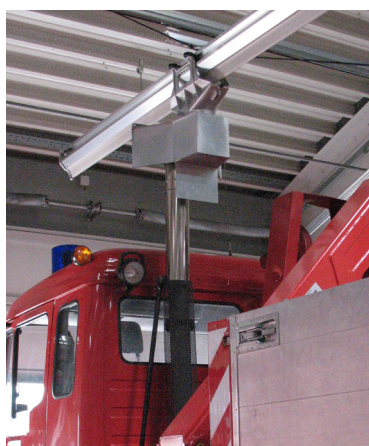
Sideways sliding extraction hood for top exhaust.
